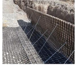
Attach the support struts, 5 large and 5 small, to each panel once the facing wrap components and geogrid are in place. It may be necessary to cut through the facing wrap to attach the struts to the panels. The reinforced soil can be placed when the struts are installed.
