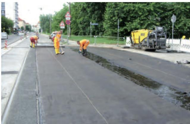
At structures such as gully holes or manhole covers SamiGrid® can be simply cut out with a knife.
