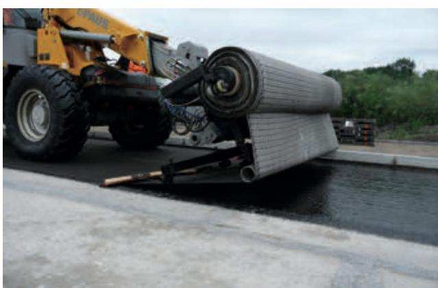
prevent it from being lifted. If several lanes are placed side by side or behind each other, overlaps shall be arranged with offsets to prevent multiple overlaps occurring at the same location.
