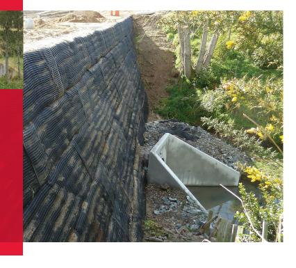
Once the backfill elevation has reached 150mm below the level of the facing, pull the facing wrap from the front of the wall back over the compacted soil. Pull the facing wrap taut and compact the final 150mm to the top of the hessian/geotextile bags. It may be necessary to stake or pin the wrap to keep it taut while backfilling. Continue the construction sequence by placing another row of geogrid and hessian/geotextile bags and repeating the construction steps.
