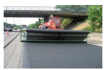
The unrolling can be undertaken with the help of a simple system, either manually, or mechanically when using wider, heavier rolls.
