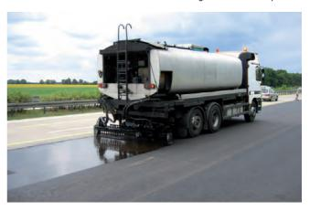
When using a 60 % bitumen content the minimum rate of emulsion (considering the residual bitumen) needs to be adjusted accordingly.
