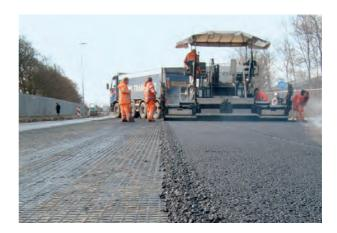
The paver and delivery vehicles should move carefully over the grid-covered surface to avoid grid displacement. Sharp turns, rapid changes in speed and hard braking should be avoided, when moving to the front of the paver. The supply vehicle in front of the paver should be driven and not pushed.
