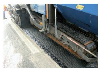
The reinforcement grid must be laid free of folds and waves. However, if a slight wave builds up in front of the paving machine, this will not detrimentally affect the performance of the reinforcement. Joints in the asphalt pavement must not coincide with overlaps in the rolls of reinforcement grid. The current technical requirements for the compaction of asphalt layers must be observed when using HaTelit®.
