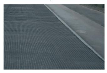
The surface should be prepared in accordance with recognised technical standards to ensure a good bond between the asphalt layers; it should be dry, clean and free of loose material.
