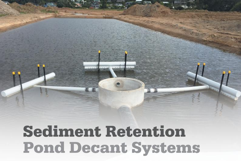
Manufactured in accordance with the Auckland Regional Council TP90, the Cirtex T-Bar Decant System is a quick and easy solution for dewatering Sediment Retention Ponds and Decanting Earth Bunds.
