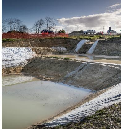
The general design approach is to create an impoundment of sufficient volume to capture a significant proportion of the design runoff event, and to provide stilling conditions which promote the settling of suspended sediment.
