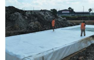
supplied a PVC liner which was wrapped on site. The RainSmart system was successfully installed and commissioned with support from the Cirtex site support team.
