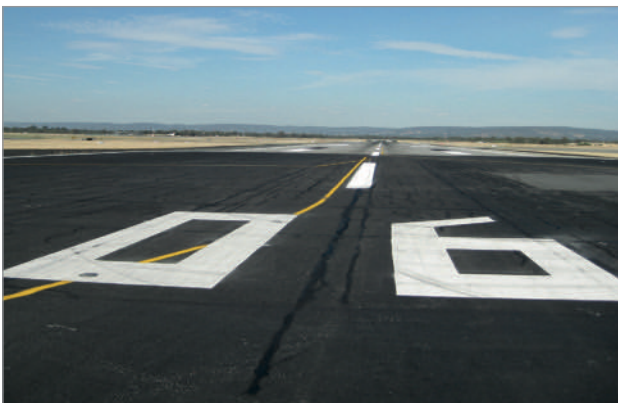
Pavement condition in 2009 prior to rehabilitation
