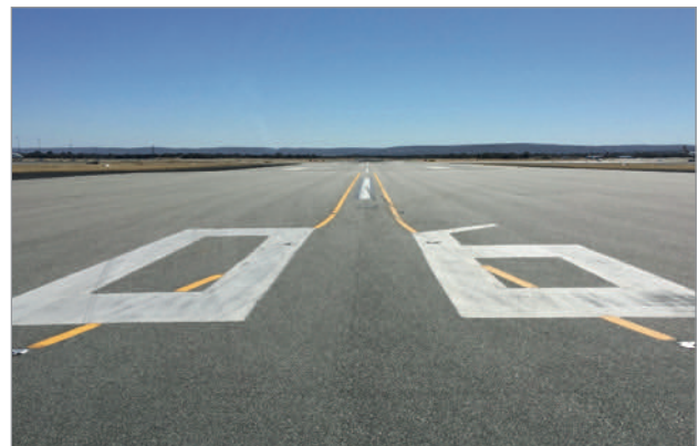
Situation approx. 10 years after rehabilitation with HaTelit C 40/17
