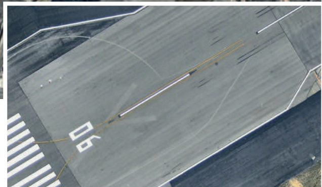
Aerial Photo of the Runway 06 Threshold in 2020
