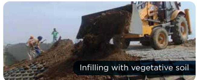
Soil fills should be lightly hand-tamped with a mechanical tamper. In case of concrete (grade shall be as specified on the drawing), the infill should overtop StrataWeb® just adequate to trowel smooth without the rim of StrataWeb® being visible.
