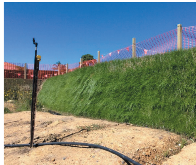
Post installation - implementation of hydro-seeding and mulching
